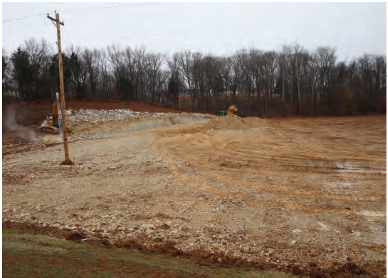
Crews have been working for weeks to clear and level the area for the new ball field.
